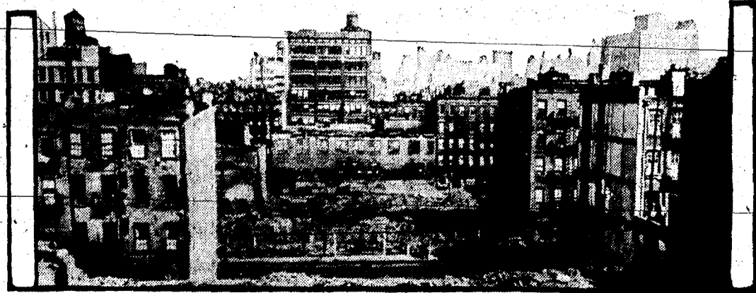
Demolition of ninety-one old houses in the Hell's Kitchen district, to make way for the Manhattan approach to the Midtown tunnel has been started. The work involves the razing of structures from Thirty-fourth street to Forty-second street, between Ninth and Tenth avenues.
