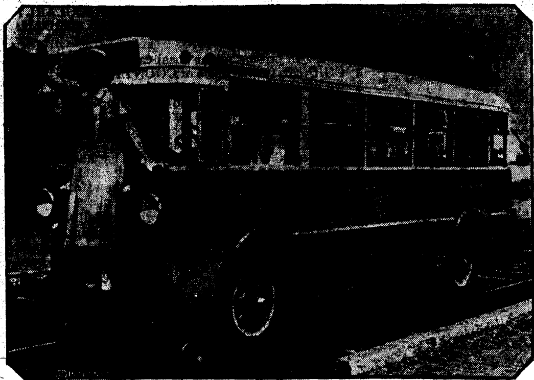
This railroad coach that can leave the rails and go wandering about the country like a stray auto was demonstrated by the Illinois Central railway. It has pneumatic tires for use on roads and pavements and is fitted with auxiliary wheels for traveling on railroad tracks.
