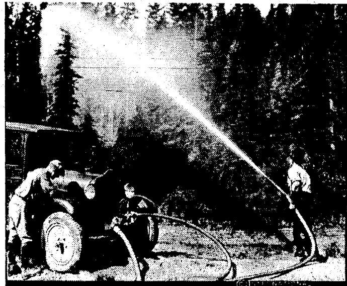
Modern firefighting apparatus is introduced in remote mountain districts of British Columbia to combat the blazes that have proved so disastrous in the past. A number of these light trucks have been put into service by the Canadian government's parks department. The motor engine is used to operate the automatic pumps which can throw a powerful stream upon the blazing bush.
