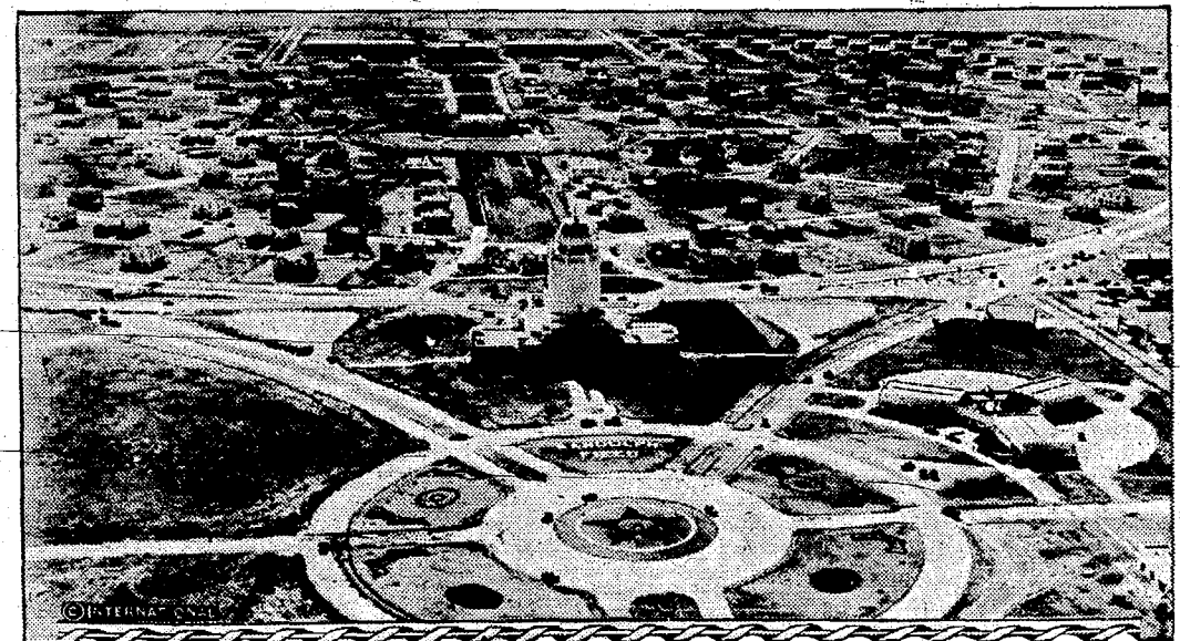
Known as "the West Point of the Air," the new Randolph field, 16 miles northeast of San Antonio, stretches like a model city before the camera eye in this aerial photograph. The "field" will include 500 buildings surrounded by flying fields for the use of the 500 planes and 3,500 pupils and instructors who can be accommodated.
