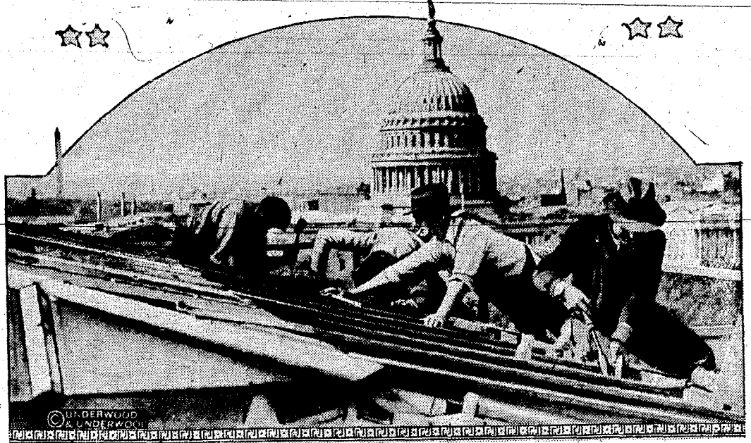
The famous gilded roof and dome of the Library of Congress, which have gleamed in the sun since 1897, having lost their glitter, and, more important, their rain-repelling abilities, are being replaced by a duller but more substantial covering of sheet copper. The photograph shows some of the workmen putting the finishing touches on the roof.
