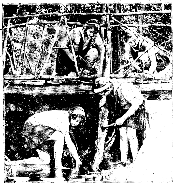
Campfire Girls repairing the damage caused by beavers to the rustic bridge made by them across the brook at their camp in Harriman State park, New York. Industrious beavers ate away the living trees which formed the natural supports at the land ends of the bridge.
