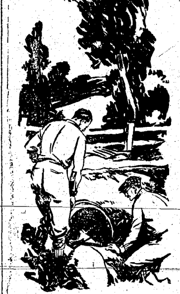
Made an Examination of the Culvert.
