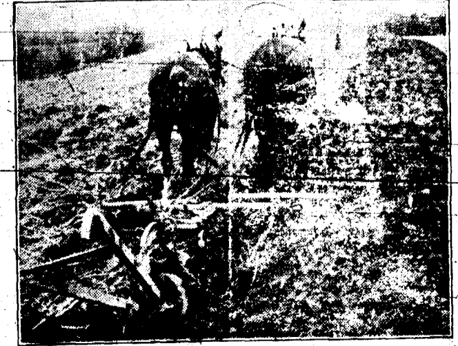
For years farmers have attached heavy chains, as illustrated, to plows to get trash well plowed under. The practice is especially useful now in burying larvae of the European corn borer which winter over in cornstalks. Long wires properly attached to the plow will do the same thing.
