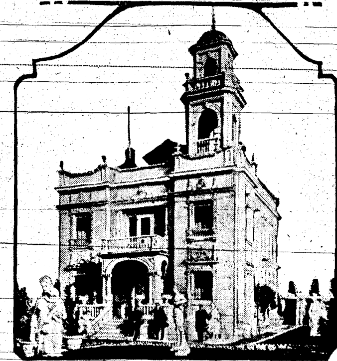
This Atlantic City residence of Capt. John L. Young, owner of the famous million dollar pier at the New Jersey seaside resort, has an address like no other in the world. It is officially recognized by the United States post office authorities as "No. 1, Atlantic Ocean."
