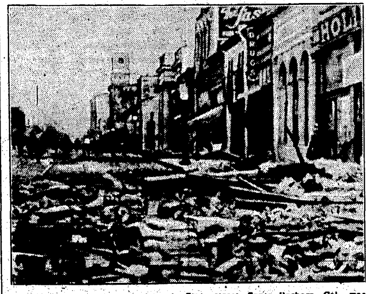
This picture of the wreckage in State street, Santa Barbara, Cal., was made immediately after the first earthquake shocks that shattered that beautiful city. It was transmitted over the wires of the American Telegraph and Telephone company.
