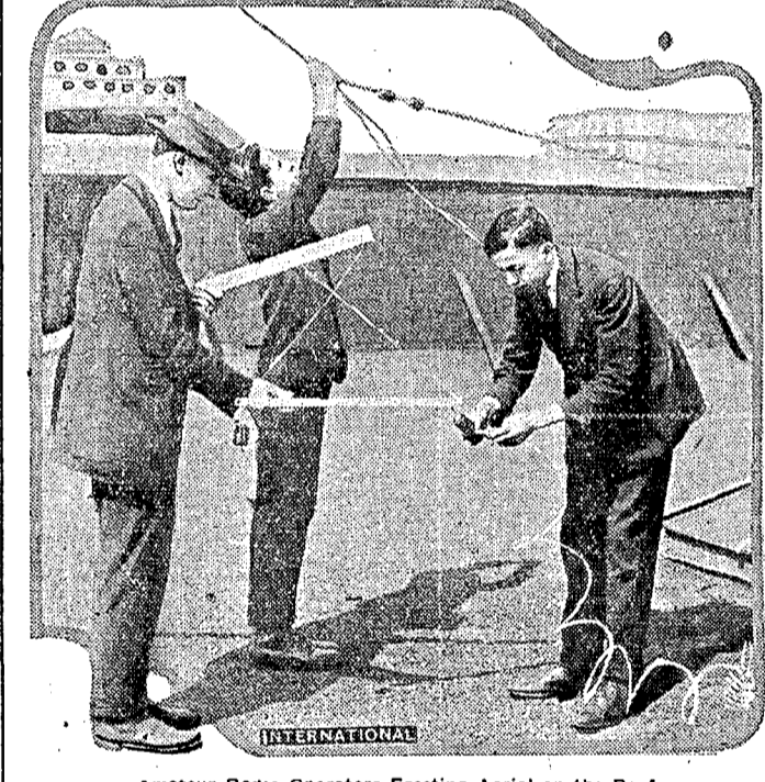
Amateur Radio Operators Erecting Aerial on the Roof.
