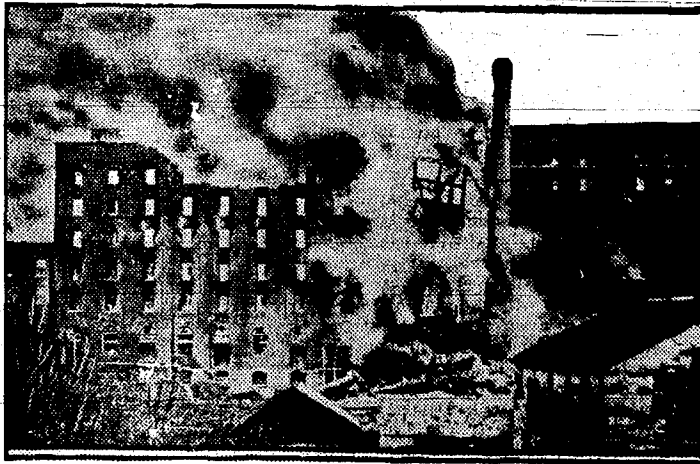
Destruction of a Mill Caused by a Dust Explosion.
