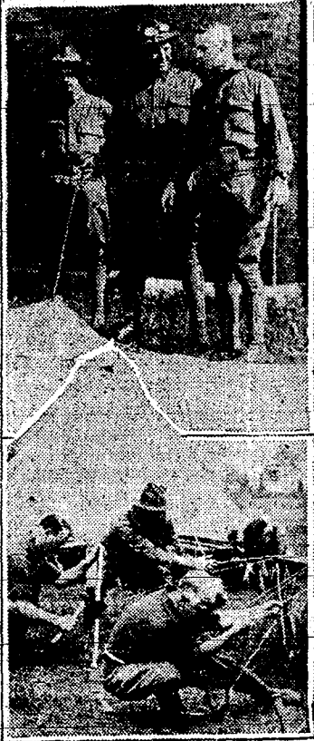
PLATTSBURG BOOKIES—BELOW, ERECTING TENT.
