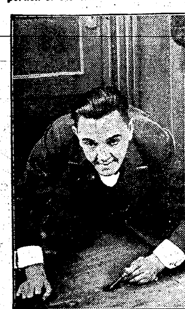
Traces the Telephone Circuits.
