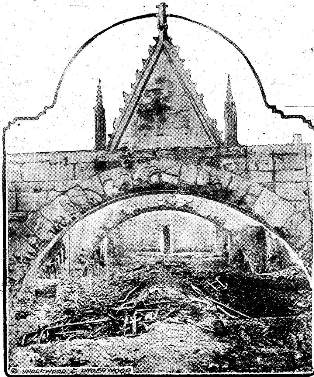
Photo shows damage done to the roof of Rheims Cathedral by the German shells. The photograph was taken from one of the surrounding towers.
