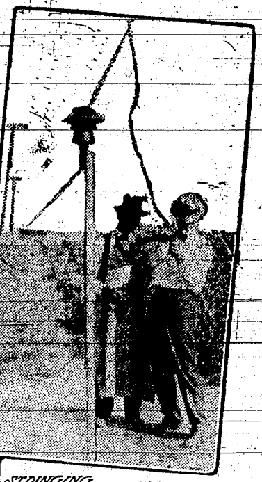
STRINGING WIRES ON FARM
