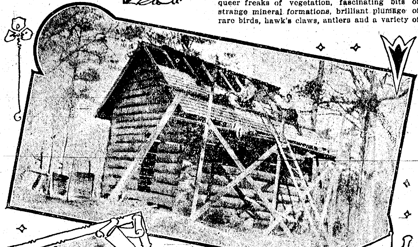
THE 5,000 1/4-INCH ROOFING BOARDS ARE SPLIT FROM 18-INCH LOG LENGTHS
