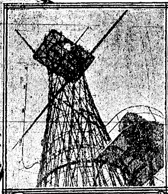
NEW STYLE MAST FROM BELOW
