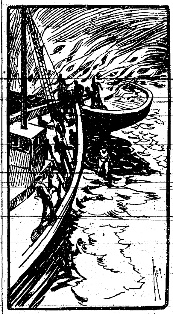
Rammed the Burning Vessel.
