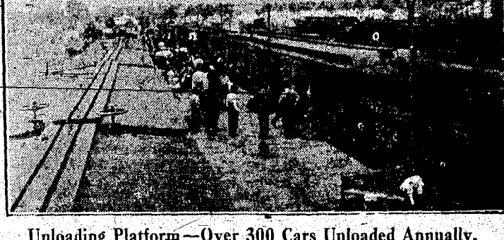
Unloading Platform—Over 300 Cars Unloaded Annually.
