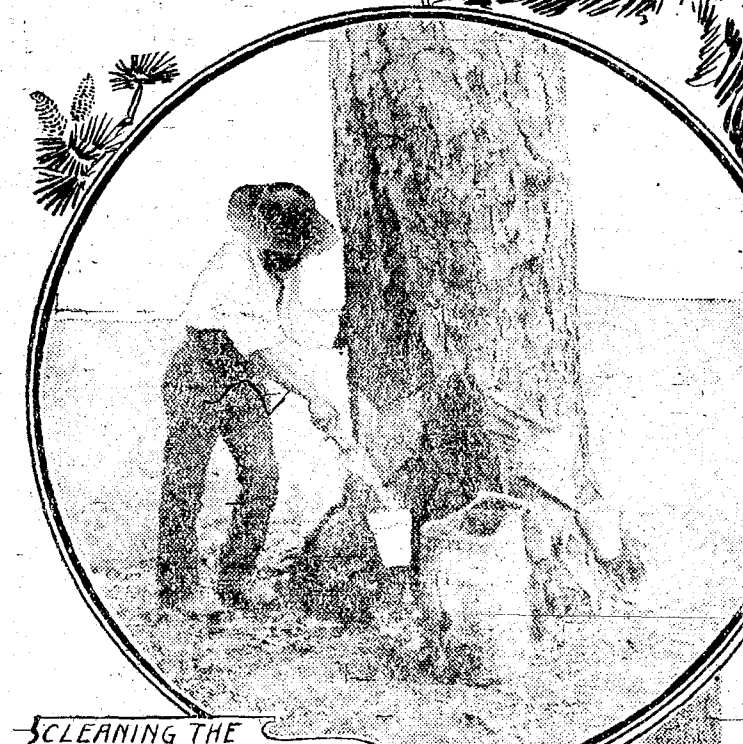
CLEANING THE GUTTERS PREPARATORY TO DIPPING
