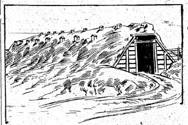
Cur illustration shows a form storage used in Colorado for storing ranged at each side of the driveway potatoes or roots. It is a dugoutfinished up like a cellar and roofed over. Ventilators are put in to give The picture shows the outer construction well. These dugouts are made large enough so that a team can be driven through them, and
