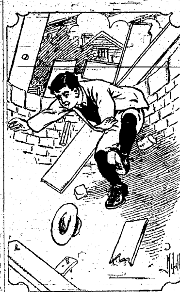
He Plunged Headlong Through the Rotten Boards.
