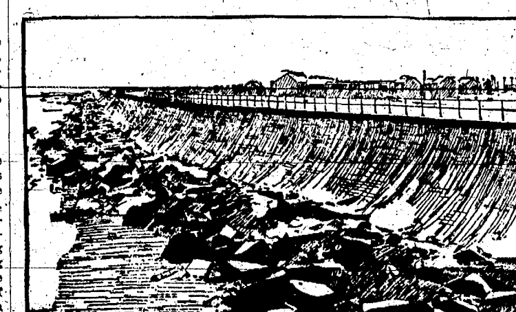
A Portion of the Gigantic Sea-Wall Being Built for the Protection of the City of Galveston.
