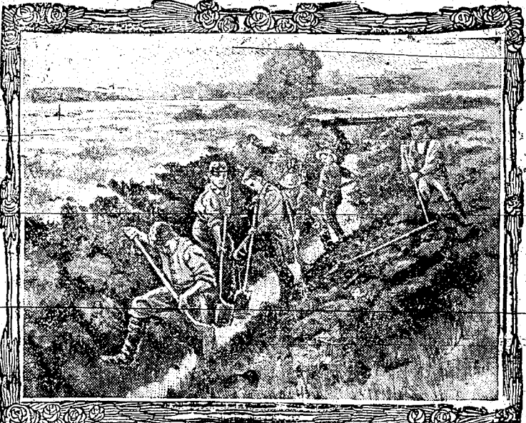
STUDENTS CLEANING OUT A DRAIN AT WINONA.
