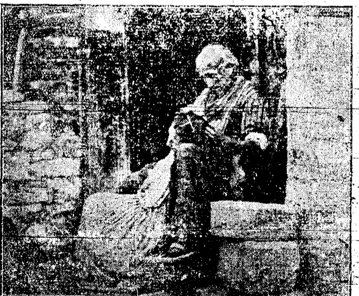
Toilet in Doorway.
