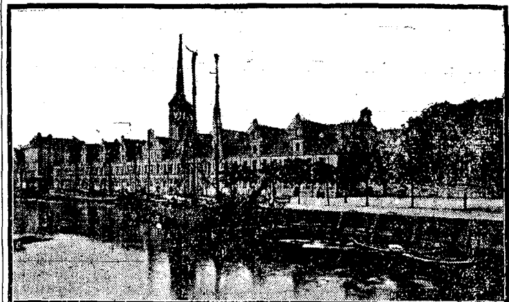
Along the Wharf.
